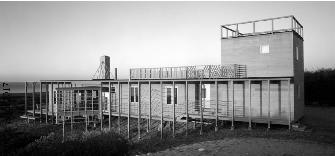
Figure 7.15: Completed project of Steven Holl's House at Martha's Vineyard
